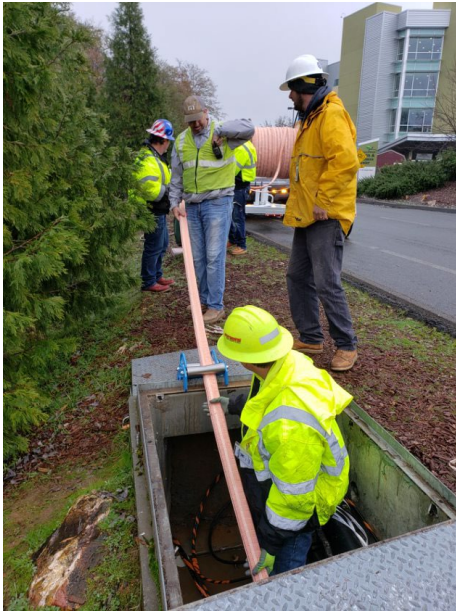
Our crew at work on a project to deliver redundant fiber to the Red Hawk Casino in Shingle Springs.
