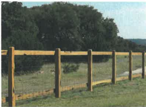
OPEN SPACE: Wood Frame Hog Wire
