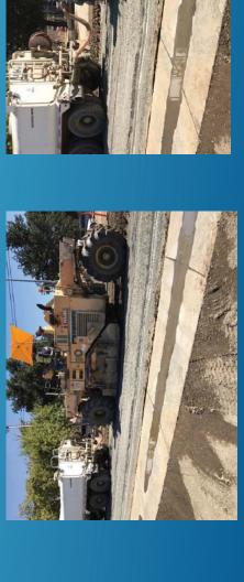
FULL DEPTH RECLAMATION (FDR) – PLACEMENT OF LIME (CEMENT) ONTO THE BASE OF THE ASPHAL)
