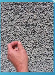
CAPE SEAL – COMBINATION OF A CHIP SEAL AND SLURRY SEAL
