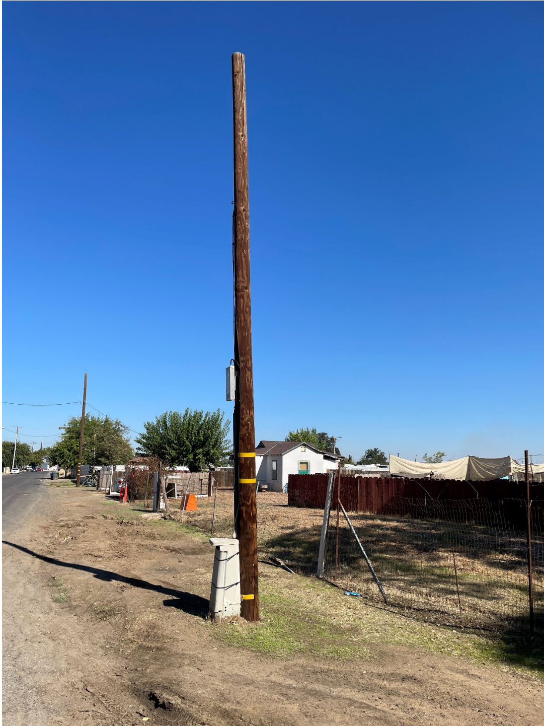
Canal Street looking north towards Childs Ave from the southerly portion of the project.
