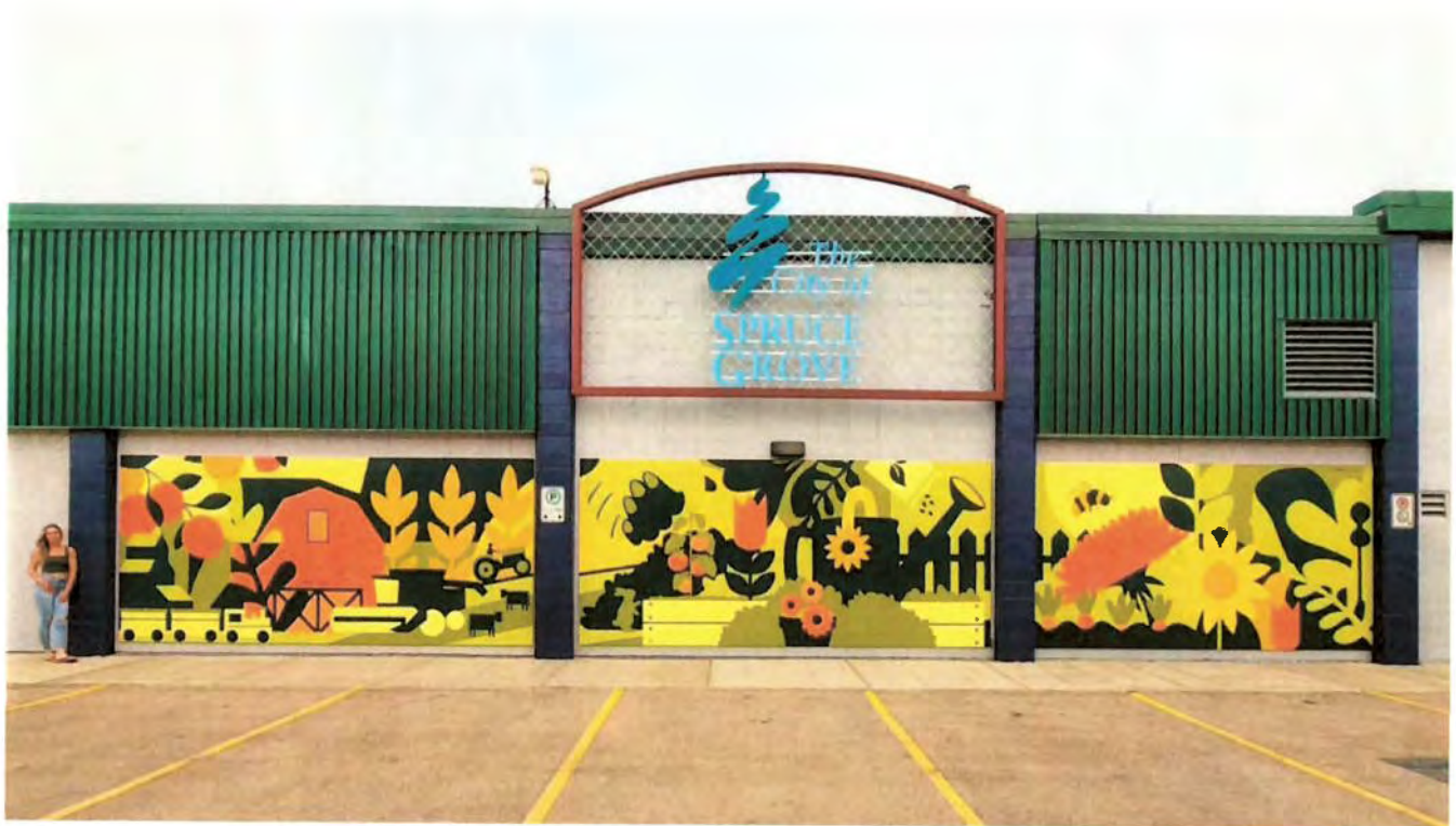
Spruce Grove Arena
