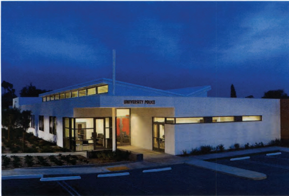
CSU Fullerton Police Facility
