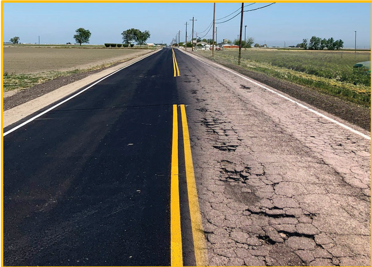
Westside Regional Project: Henry Miller Ave Reconstruction Project, Phase 1 (Merged photo: Before reconstruction on the right, after reconstruction on the left)
