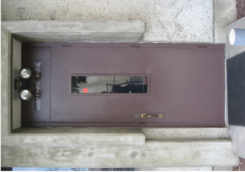
Exterior doors without 24" side clearance - concrete portico interference
