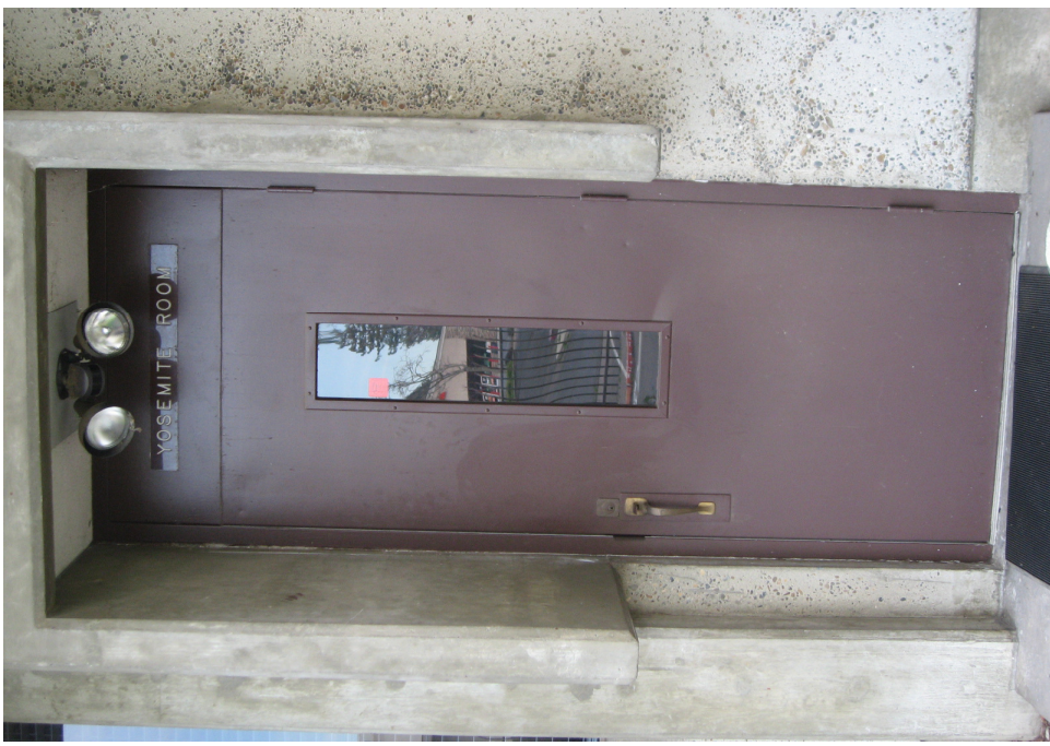
Interior doors without 18" push side clearance
