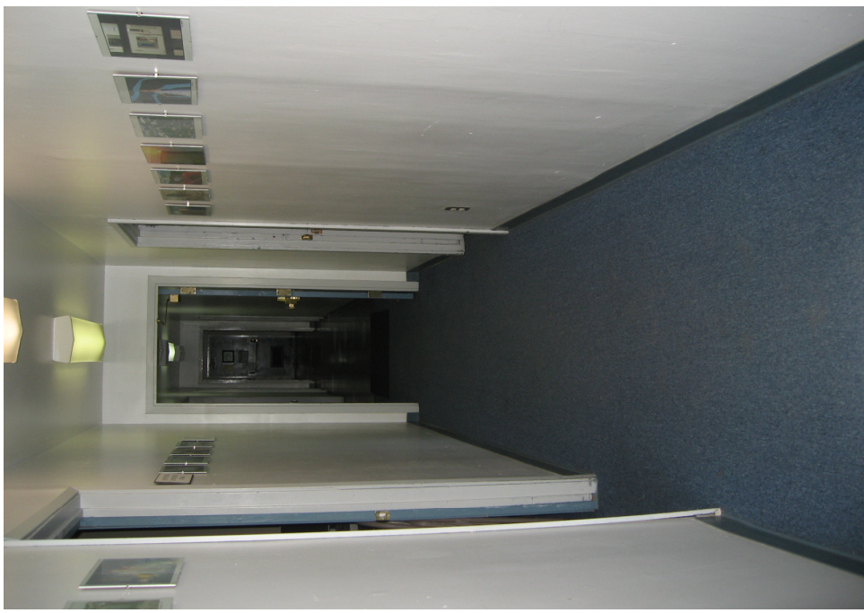
Interior doors without 18" push side clearance
