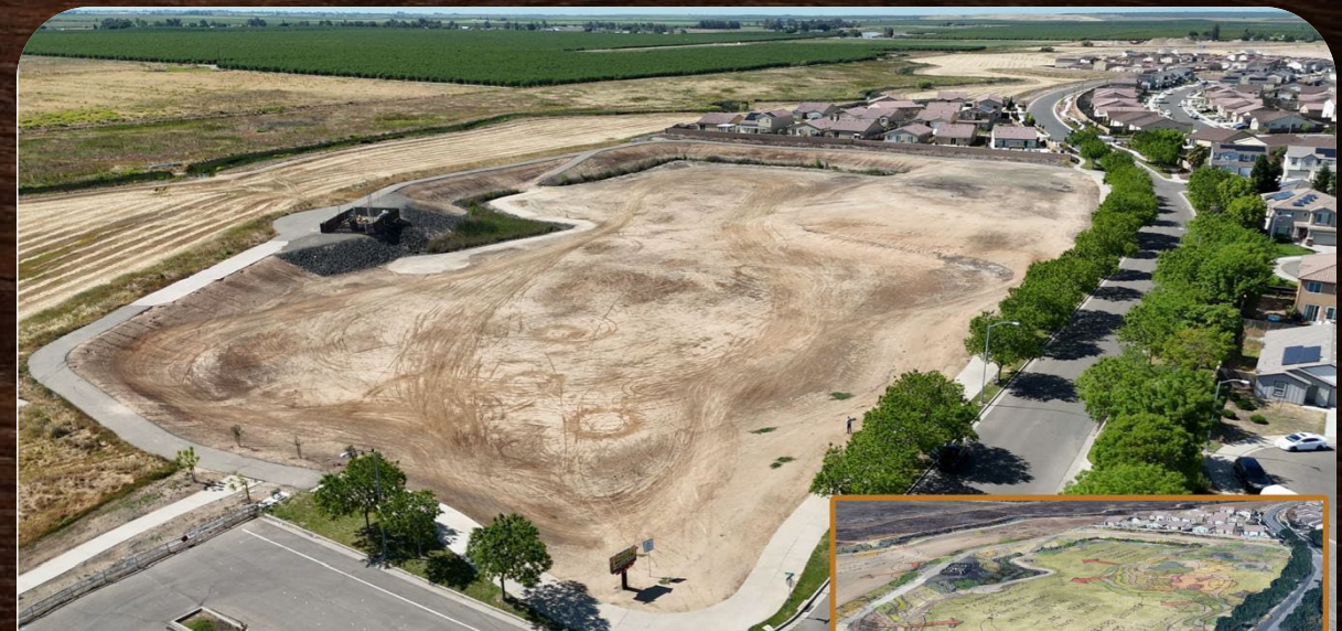
NORTHWEST - DRONE IMAGE
