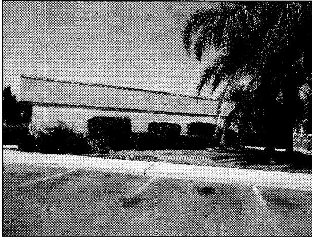
MODULAR OFFICE BUILDING – EASTERN ELEVATION
