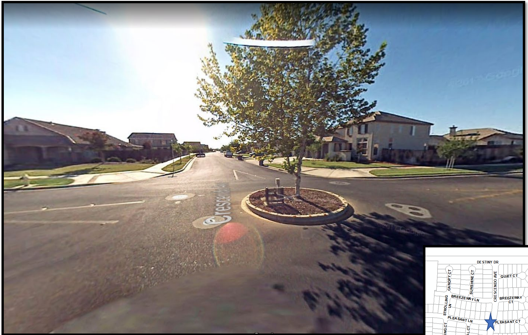
Intersection of Crescendo Avenue and Pleasant Lane/Court
