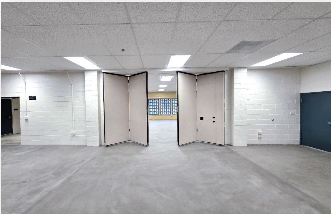
Interior Divider to Separate two Multi-Purpose Areas
