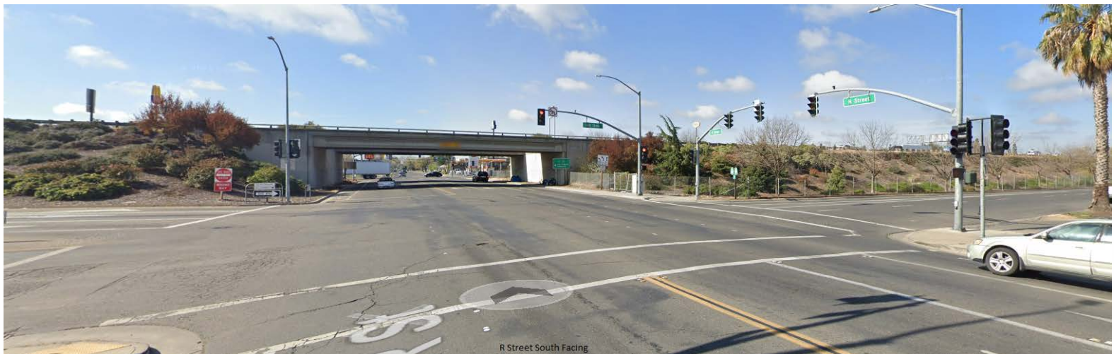
R Street South Facing
