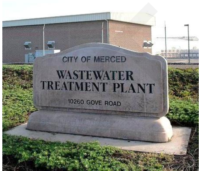
Merced Wastewater Treatment Facility
