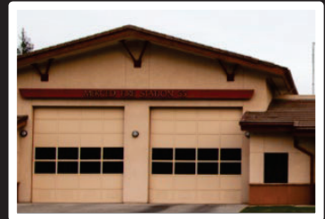
Station 55 (2006 - 14 Years Old) 3520 North Parsons Avenue
