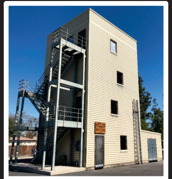
Training Tower (2004 – 16 Years Old) 99 East 16 th Street
