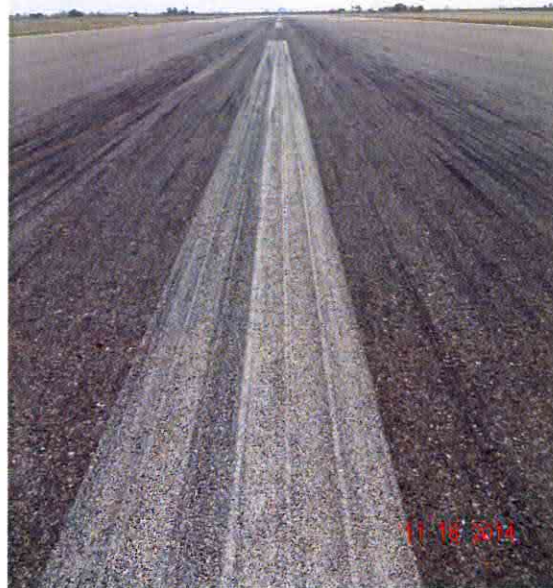
Faded Runway Centerline
