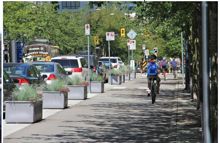
Figure 18: Class IV Bikeway with Permanent Planters as Separation
