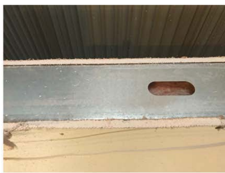
Steel interior studs and fire-rated drywall
