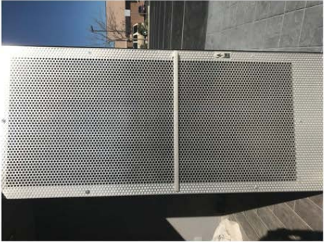
Custom steel security mesh on all doors and windows
