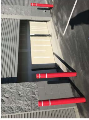
Bollards (crash posts) in parking lot and behind roll-up doors
