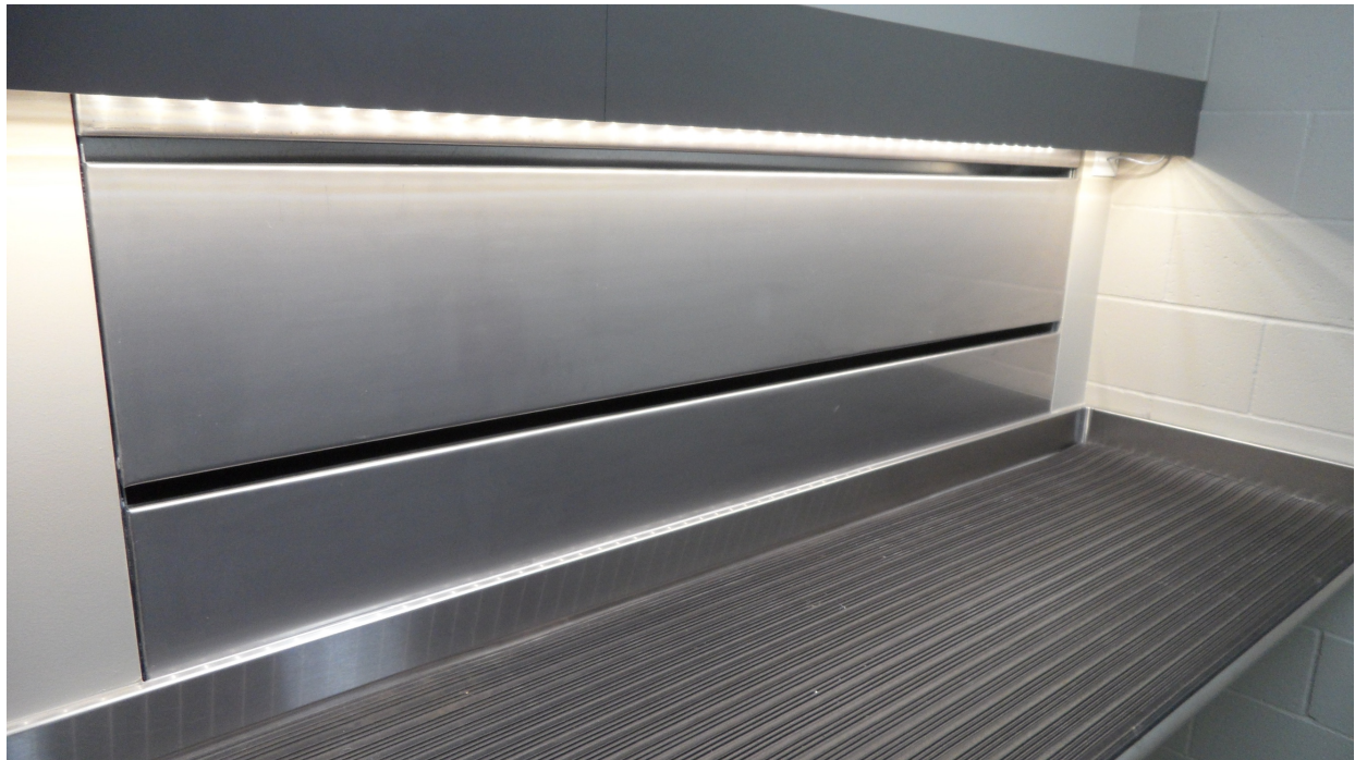
a weapons maintenance counter with lateral exhaust
