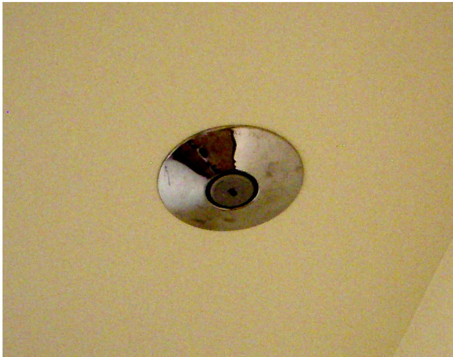
a suicide-resistant recessed sprinkler head
