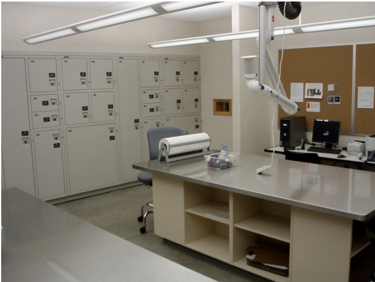
officer's evidence processing / bag & tag room shown w/ task exhauster & evidence lockers
