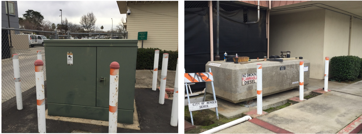
Unprotected exposed electrical service and emergency generator fuel tank.
