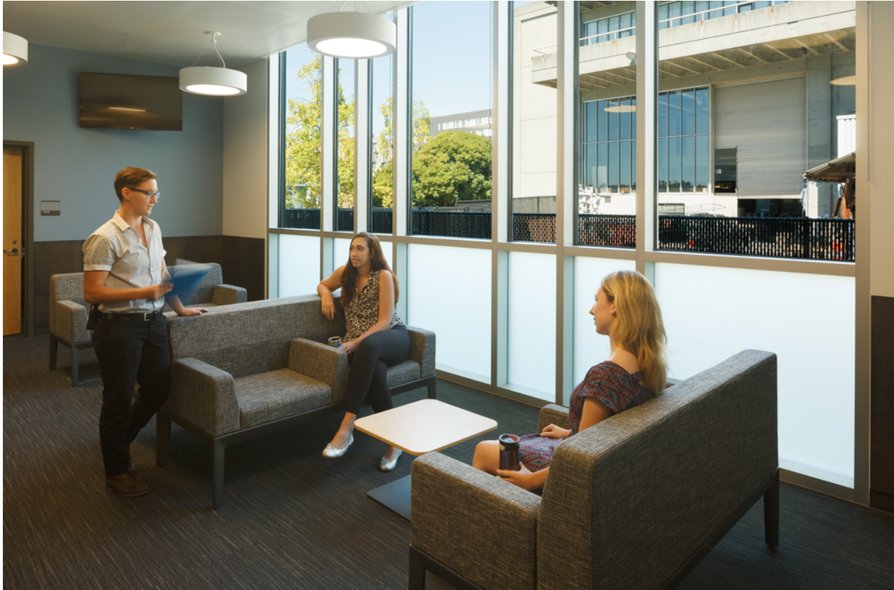
glazing shown lower than 48" is UL® ballistic rated
