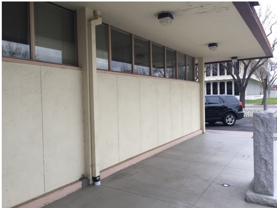
Building exterior with stucco panels covering over window wall behind.
