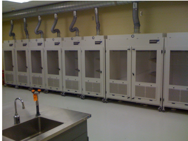
refrigerated biological evidence drop lockers and drying chambers
