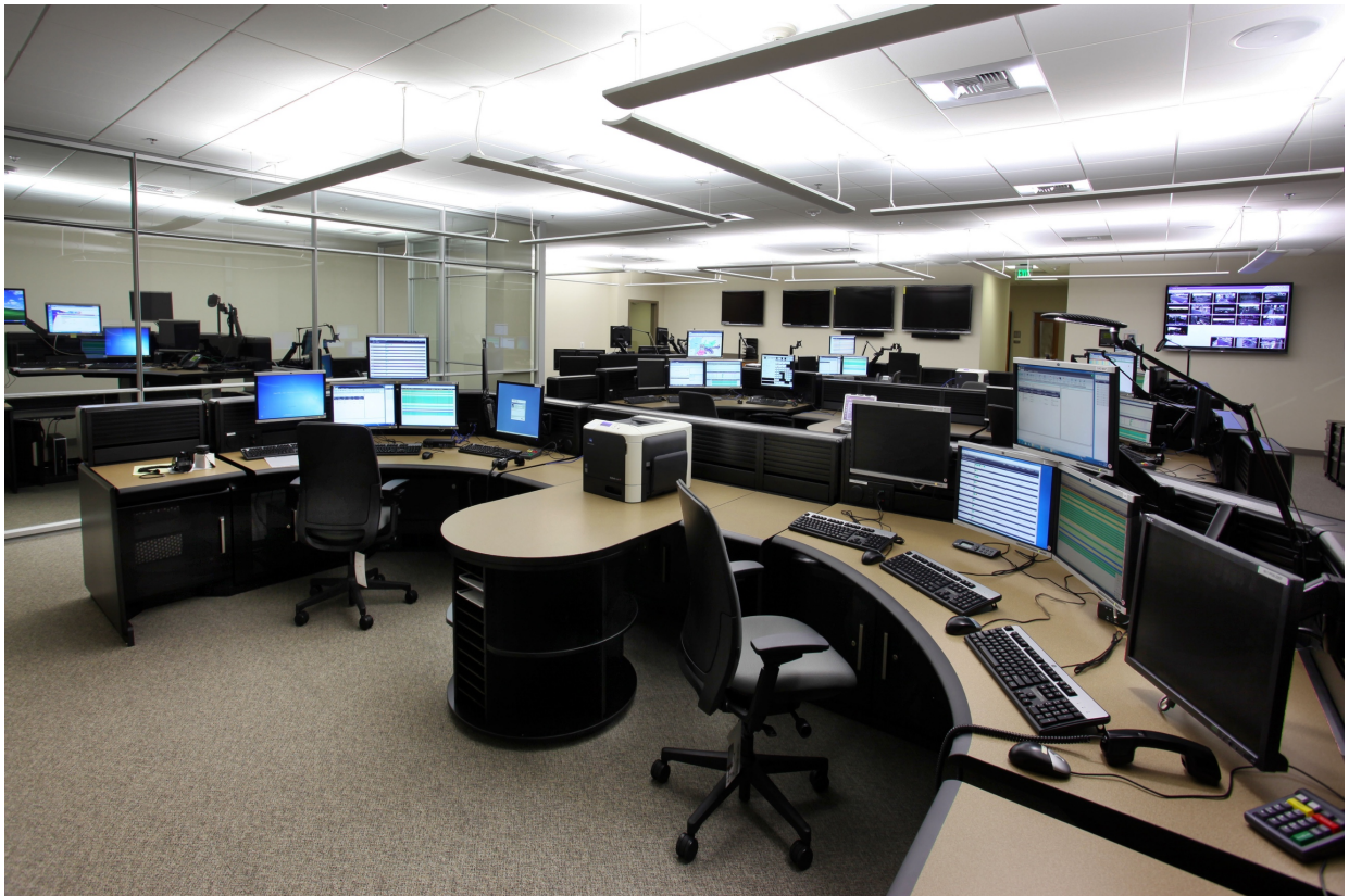
Pendant Mounted Indirect Ambient and Console Based Task Lighting
