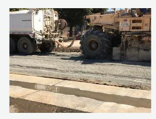
FULL DEPTH RECLAMATION (FDR) – PULVERIZE IN-PLACE ADDITION OF LIME/CEMENT
