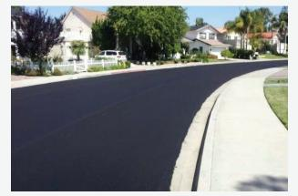
CAPE SEAL – COMBINATION OF A CHIP SEAL AND A SLURRY SEAL
