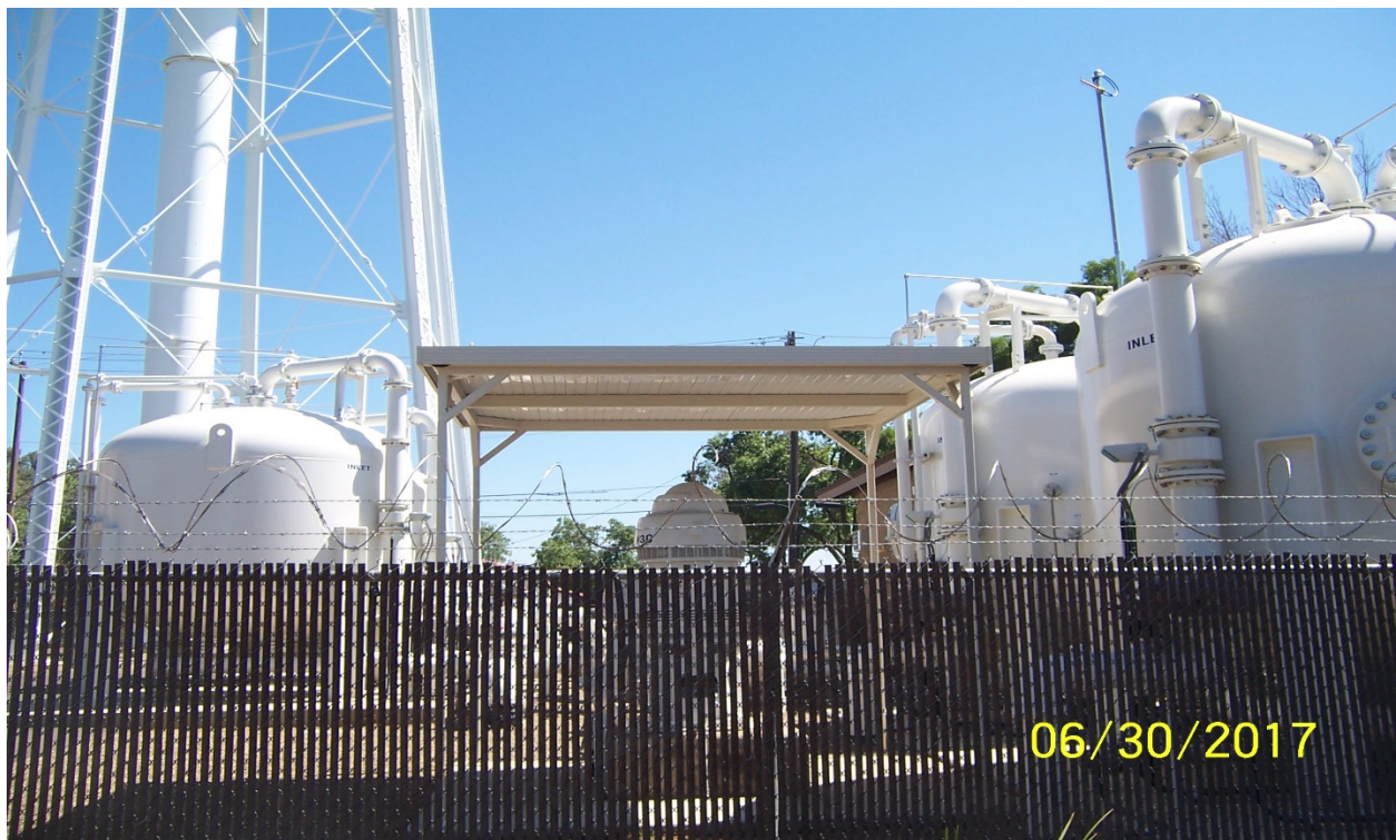
Well site 3 PCE treatment system installed.
