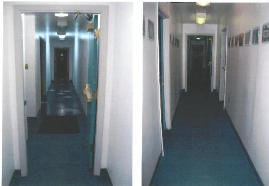
Interior doors without 18" push side clearance
