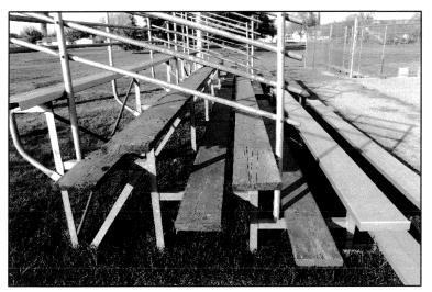
Wooden blanks have replaced sections of the aluminum bleachers that have been broken and stolen for scrap metal. Replacement parts are not available for the bleachers so staff had to make-do with the wood parts.
