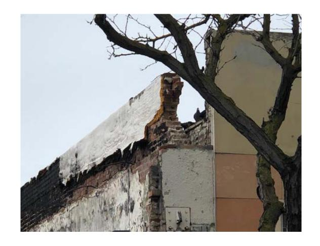
Front of parapet wall/storefront irregular and un-grouted brick work
