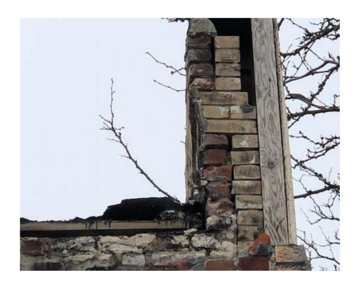
Systemic street fracture, not isolated, along the length of the parapet
